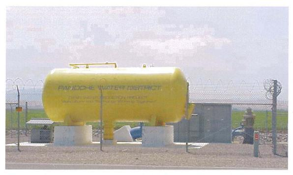
Panoche Drainage District Recirculation System Pumping Plant and Air Chamber. Districts throughout the GDA have developed drainage recirculation systems, which are a critical tool in managing drainage discharge.
