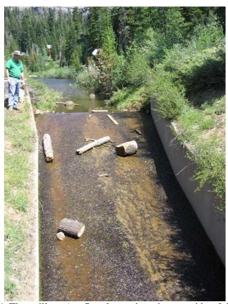
Photo 6: The spillway/outflow located on the east side of the dam.
