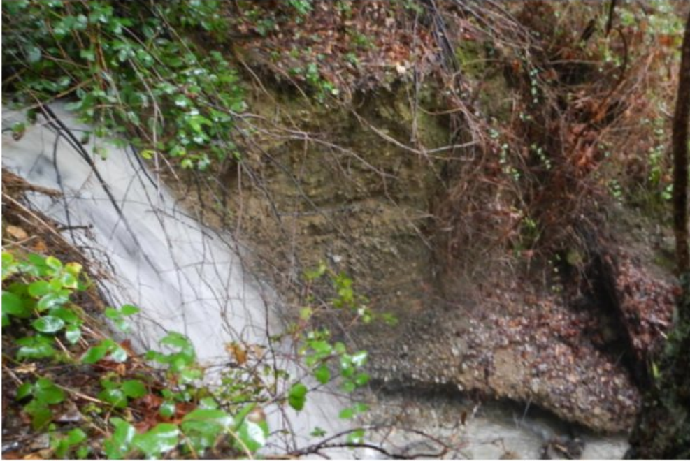
Figure 9. Gully headcut (approx. 15 feet deep) where MMR ditch leaves MMR into Irving Creek drainage.
