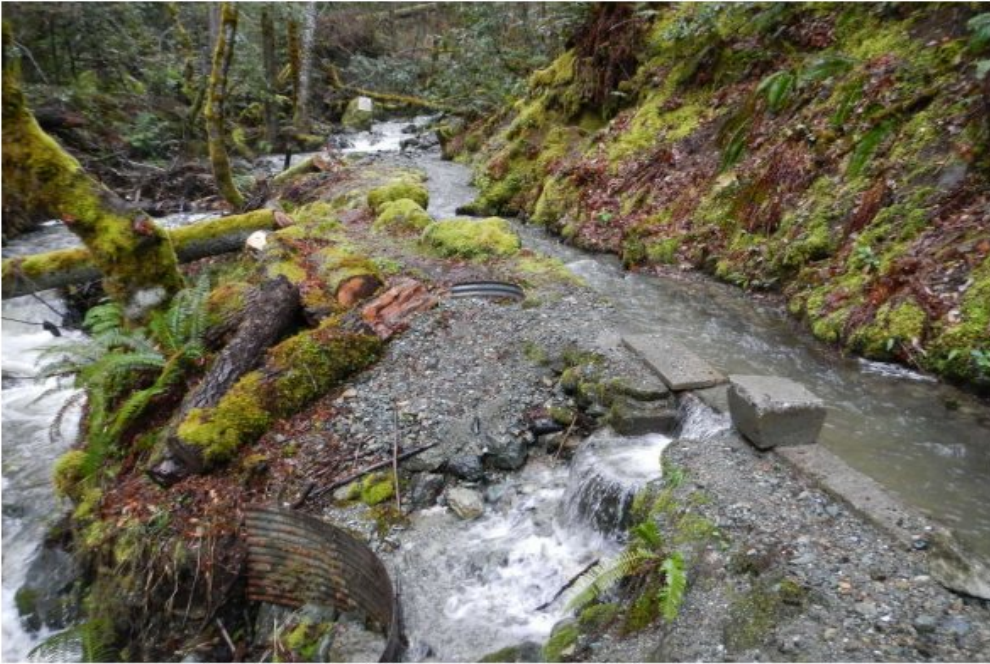
Figure 7. MMR ditch overflow just below Point of Diversion (POD).
