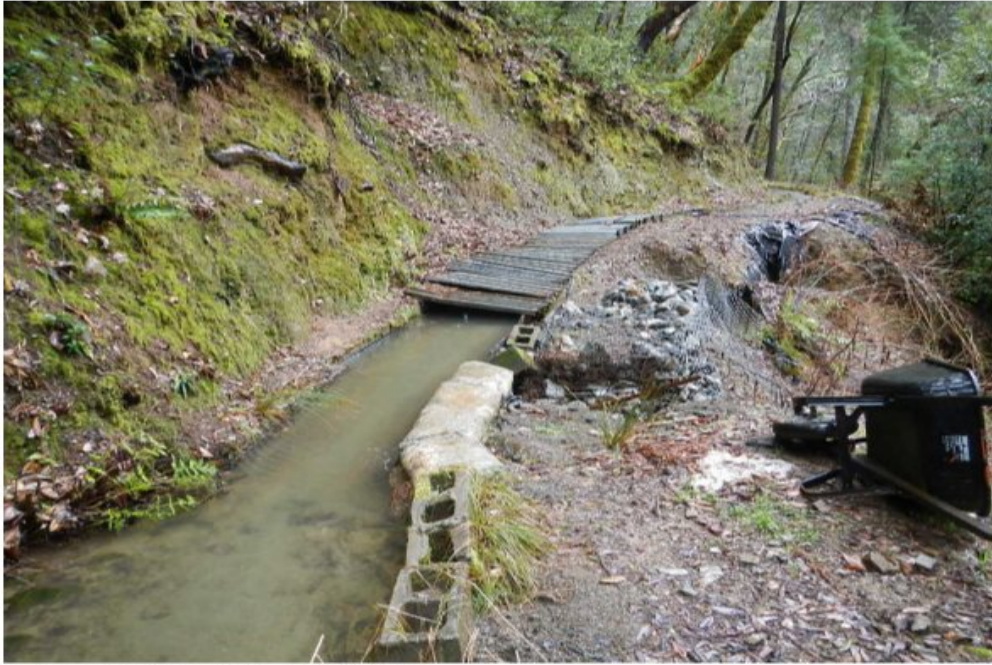
Figure 5. Repaired section of MMR ditch.
