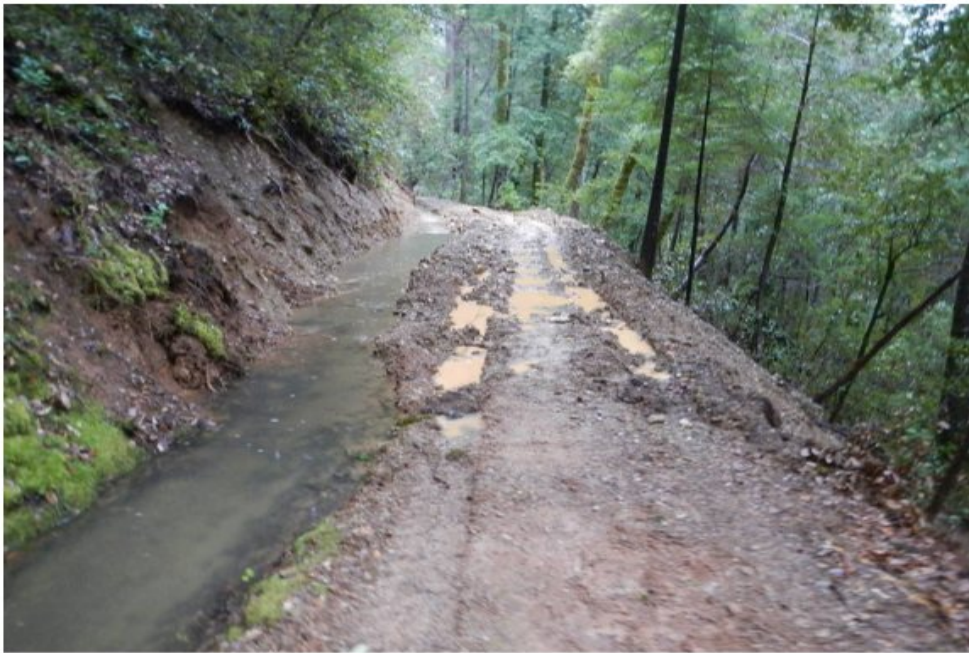
Figure 4. Recent MMR ditch repair site.
