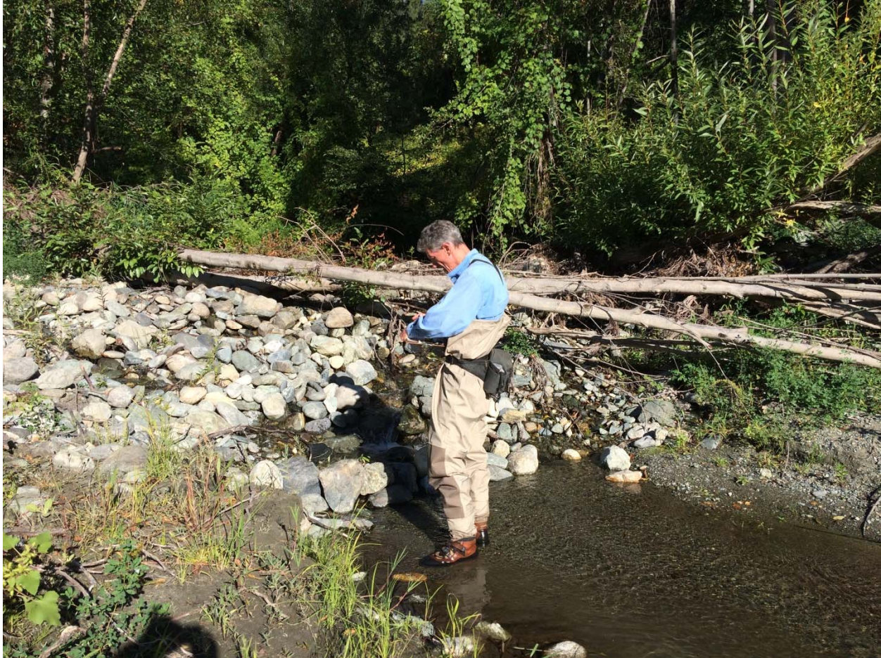
Photo 4. Rock berm at the floodplain pond outflow. I am standing in Klamath River backwater where some of Stanshaw Creek flows emerge through the rock berm to enter the Klamath. None of the flow exiting from the pond flowed out over the surface where fish could pass.
