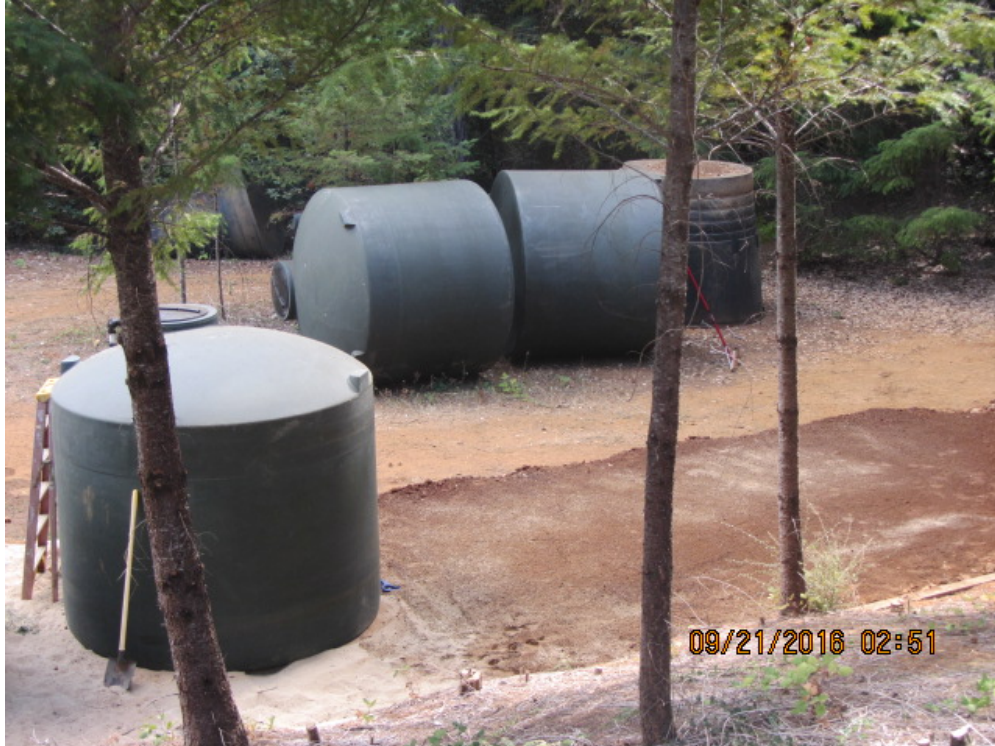
Exhibit MMR-03 Photograph #2 – Additional water storage tanks being installed
