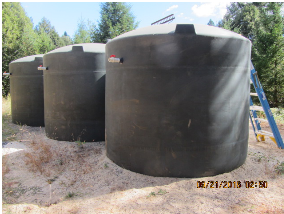
Exhibit MMR-03 Photograph #3 – Additional water tanks placed, plumbing being installed
