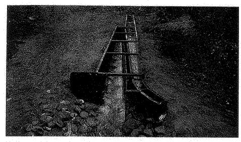
The Deep Creek diversion which supplies water to Black Lake was previously unscreened. This new two section modular Farmers Screen will ensure that resident westslope cutthroat trout, built trout, brook trout, and rainbow trout will stay in Deep Creek.
