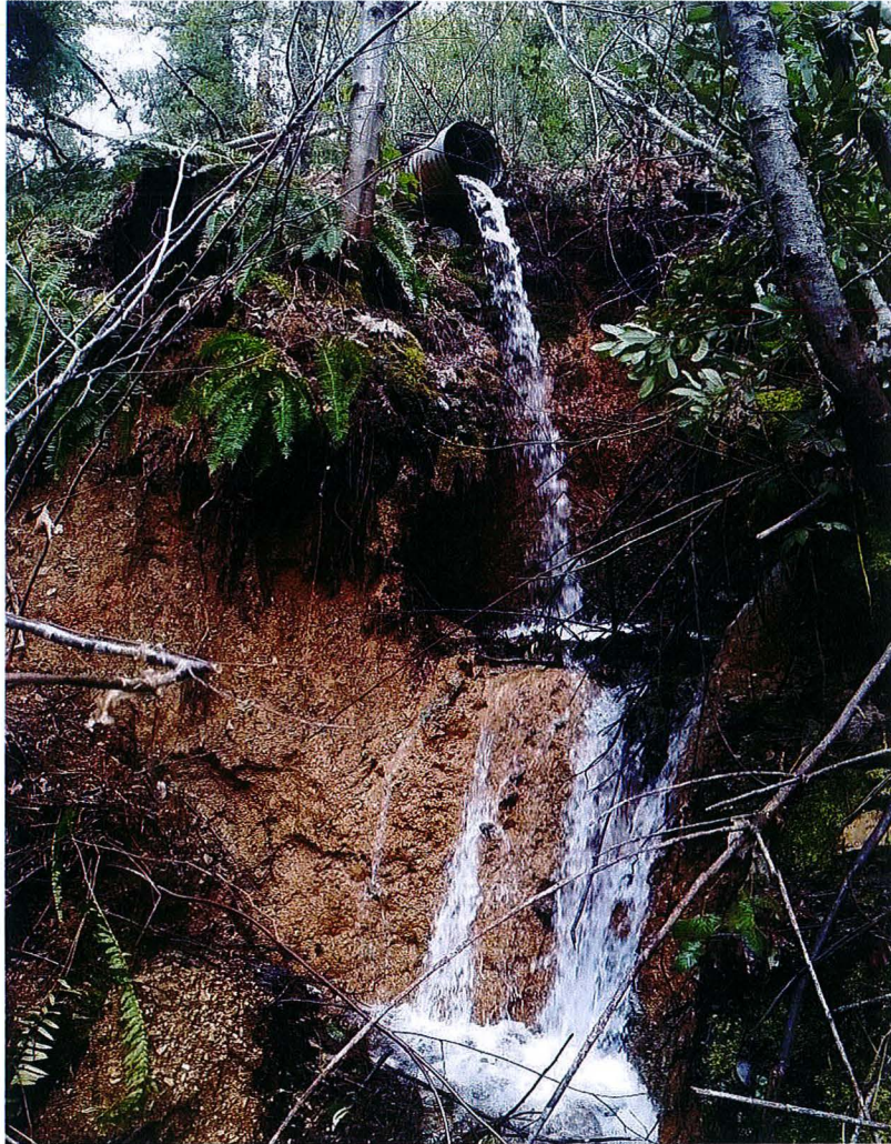
Figure 3. Upstream view of the shotgun culvert located at an unnamed tributary to Stanshaw Creek, Station 474.
