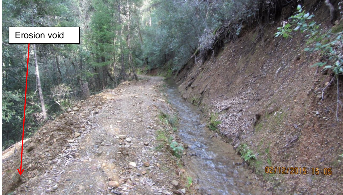
Image 21- Point 14, a cut bank that appears to have slumped in the recent past, causing water to overtop the berm and erode the berm and lower slopes. (Photo 8520 and 8521 composite)
