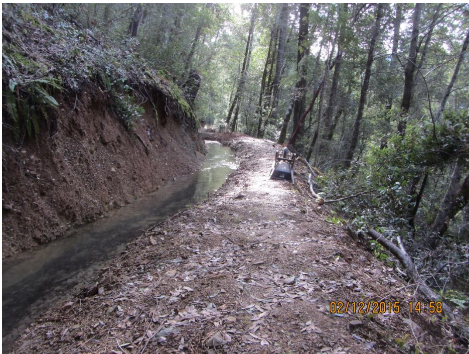
Image 20- Point 13 shows a large continuous cut bank slump that extends for approximately 220 feet. Based on my observations, it appears the cut bank slumped along this stretch over this past winter, delivering approximately 10 yds 3 of sediment into the ditch, blocking the channel, and causing water to overtop the berm
