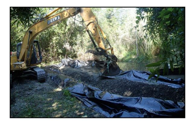
Before excavation began, a thirty foot coffer dam was constructed using 10mm plastic wrapped around washed gravel. This coffer dam excluded all mechanical construction activities from the existing pool habitat. Once construction activities were complete the dam was manually dismantled.
