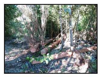
Five 30' logs with rootwads attached were locked into existing vegetation at the head of the off-channel pool, designed to redirect sediment around the project area in high flow events. The upper left and right photos show a close up, before and after, of the log placement, while the photo below shows the structure in relation to Stanshaw Creek and the off-channel habitat during winter flows.
