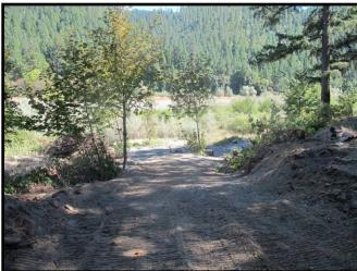
A 200 foot access road was constructed between an extisting roadway and the project site, across the Klamath River floodplain. This access road was seeded and mulched after project construction was completed. Images above left and right show the access road from the top, before and after construction. Below, the perspective show's a more complete view of the access road from the top and across the river floodplain.
