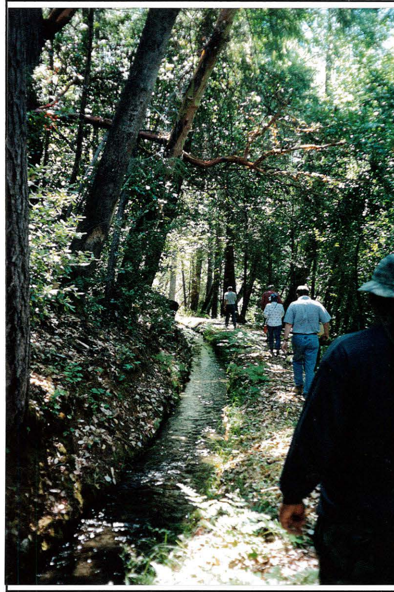
Photo 24. Looking downstream at the ditch between the water filtration point and the trash rack / penstock. The dead trout in photo 14 was found near here.
