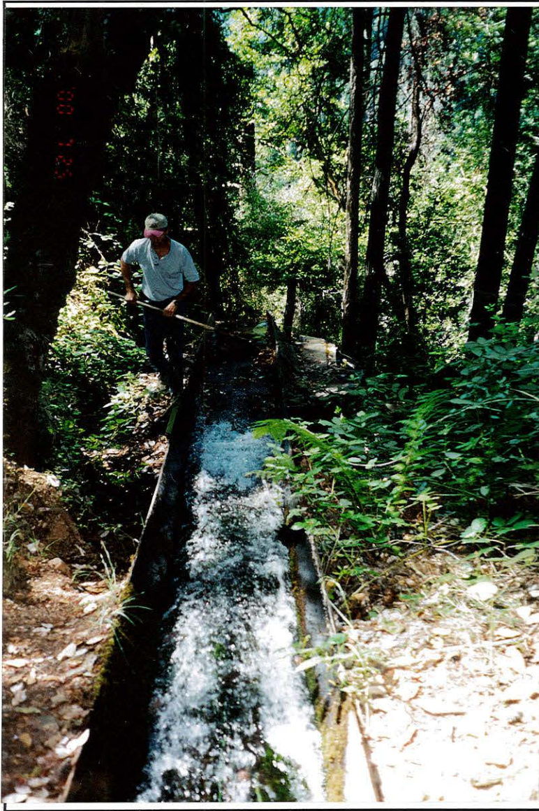
Photo 25. Mr. Cole clearing the trash rack of leaf litter. Clearing is done daily and >5 times per day during the fall. Water then enters a holding tank, thence penstock.
