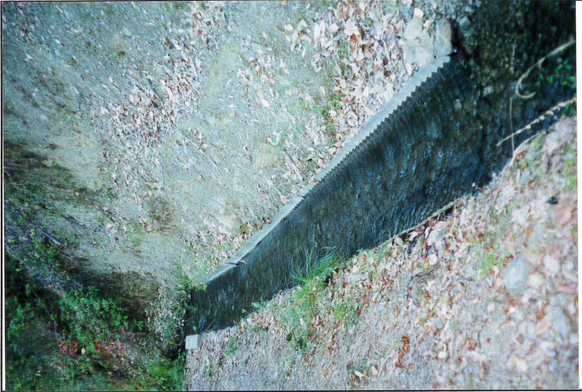
Photo 20. Half-culvert in ditch.
