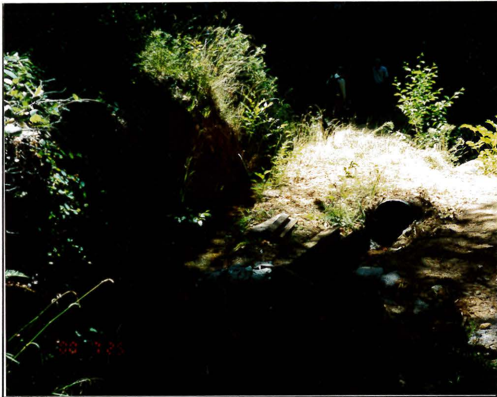
Photo 17. (left) Looking downstream at the relief structure.
