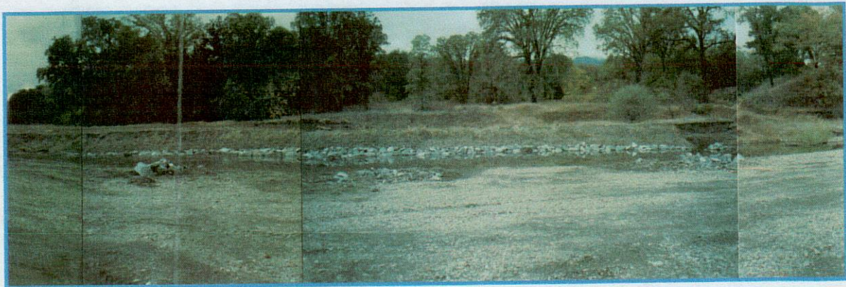
November 11, 1999. Panorama of Site 2 just after completion.
