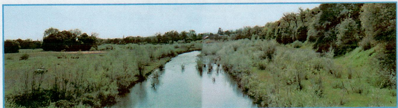
April 16, 2005. View from bridge of completed project at Site 1. Note willows line both banks.
