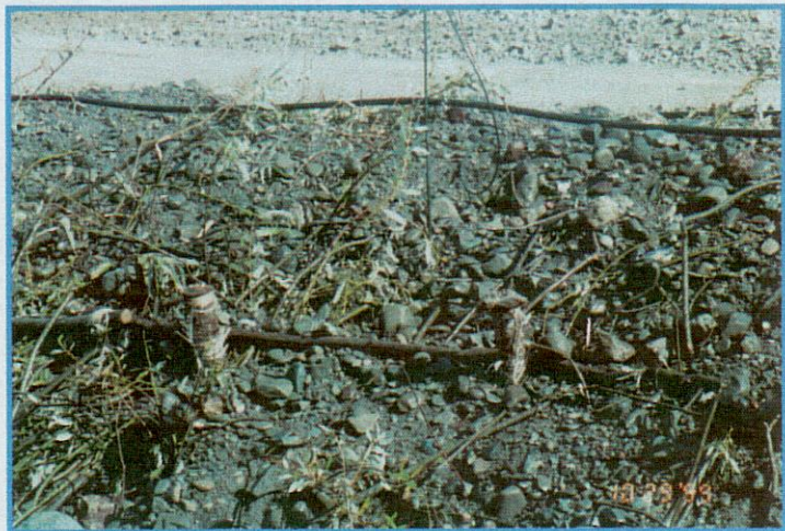
Detail of stakes anchoring willows to bank.
