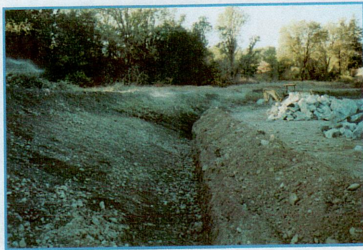
Trench for willow brush mattress.
