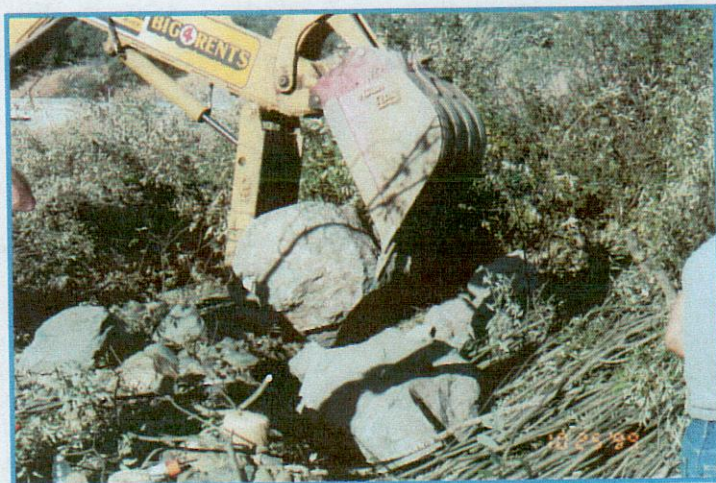
Closeup of backfilling.
