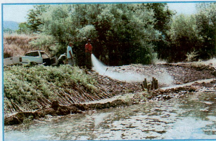
Construction of willow brush mattress.
