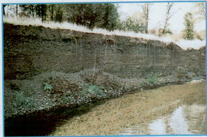
Closeup of 11-foot high vertical bank.
