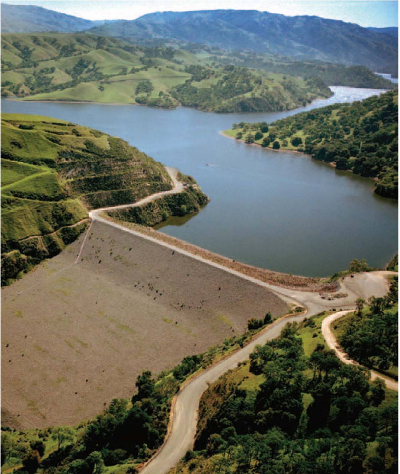
Surface storage plays an important role in California where the pattern and timing of water use does not always match the natural runoff pattern. Contra Costa Water District pumps high quality water into its Los Vaqueros Reservoir and uses it to lower salt content of water it pumps from the Delta. (DWR photo)
