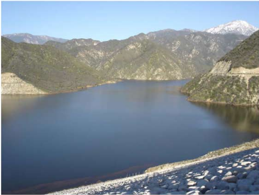
Figure 2.2-6. Seven Oaks Reservoir, March 2005
