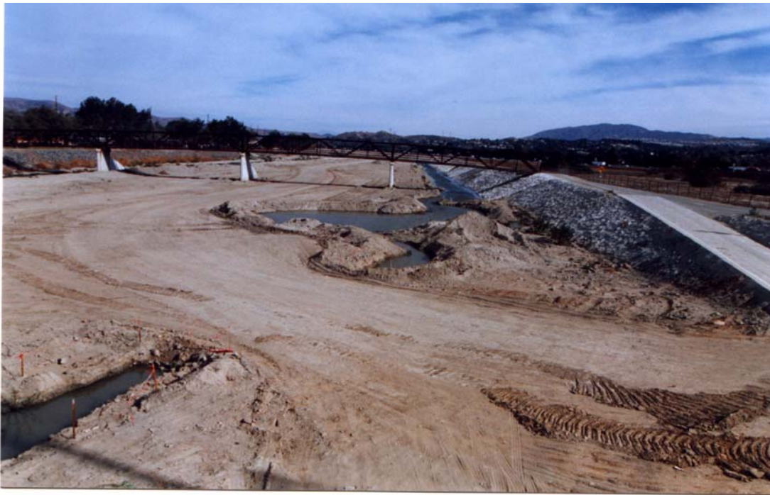
Photo 3. Santa Ana River at Imperial Highway.
