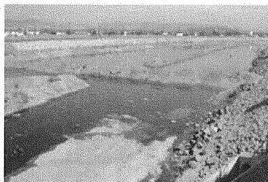
OCWD "T" and "L" levees built in recharge section of river
