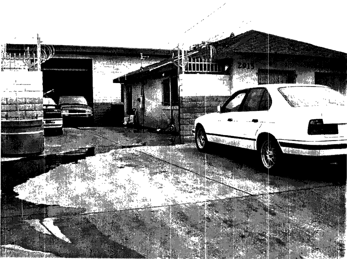
PHOTO 4. 2915 E. La Jolla Street, Anaheim, southern elevation (26 May 2004).
