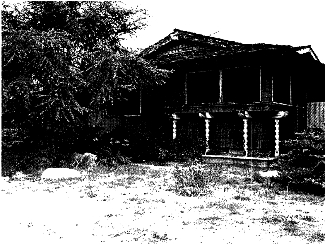
PHOTO 1. 2885 E. La Jolla Street, Anaheim, southern elevation (26 May 2004).
