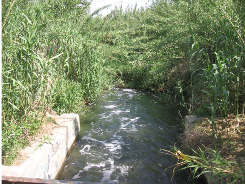
Upper end of Direct Discharge Channel (looking downstream from Structure #1).
