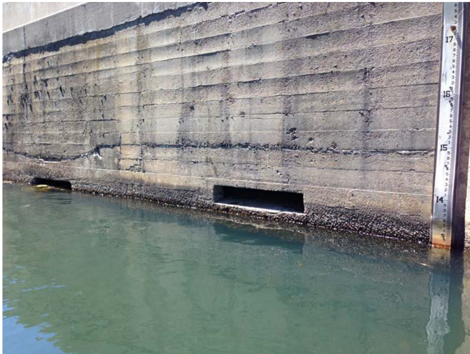
Staff gage mounted on headwall at siphon-spillway structure (photo date June 1, 2013).
