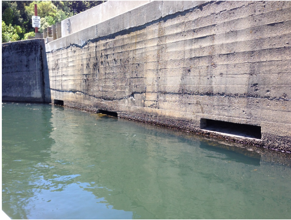
Madrone Lake Dam intake to siphon-spillway structure and staff gage (photo date June 1, 2013).
