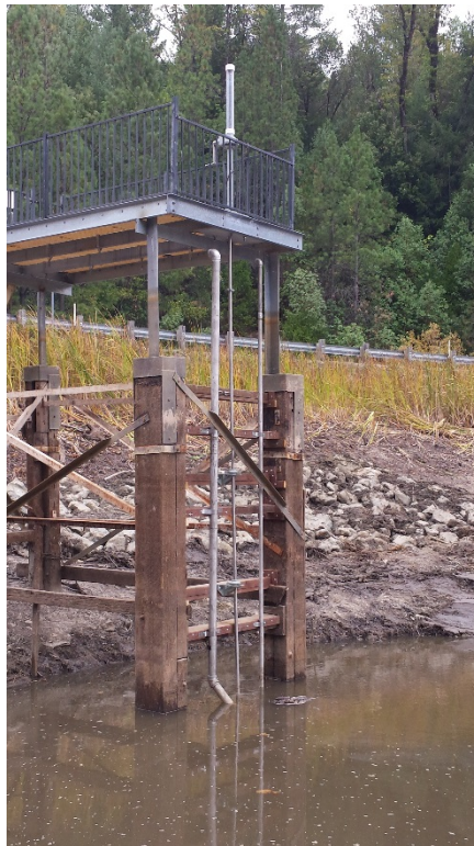
Madrone Lake Dam low-level outlet gate control (photo date October 14, 2014).
