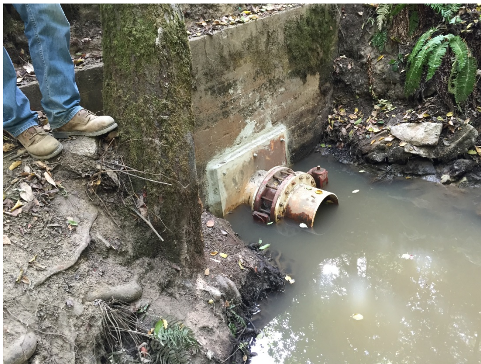
Lake Madrone Dam low-level outlet discharge on downstream side of dam, with control valve (photo date October 10, 2014).
