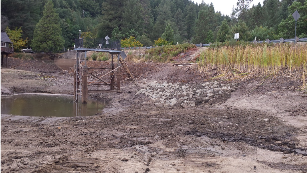
Madrone Lake Dam low-level outlet gate control; embankment dam at right, siphon-spillway structure in background (photo date October 14, 2014).
