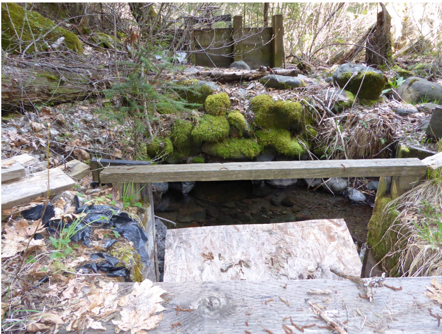
02_S-Cow-Ck_Div-43-Measurement-Box_before_Stilling_Well_installed_looking_upstream_toward_gate.JPG
