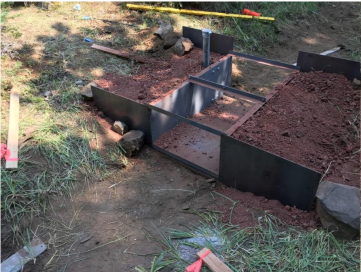
Diversion 3 Watchman Flume Installed
