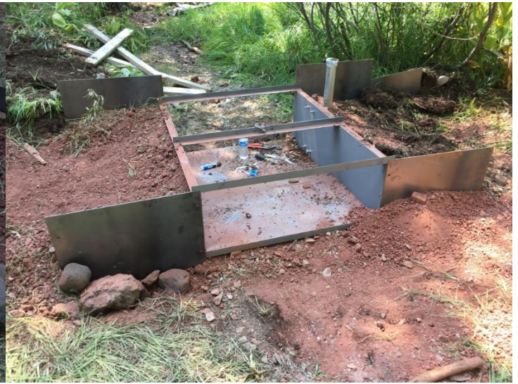
Diversion 4 Watchman Flume Installed
