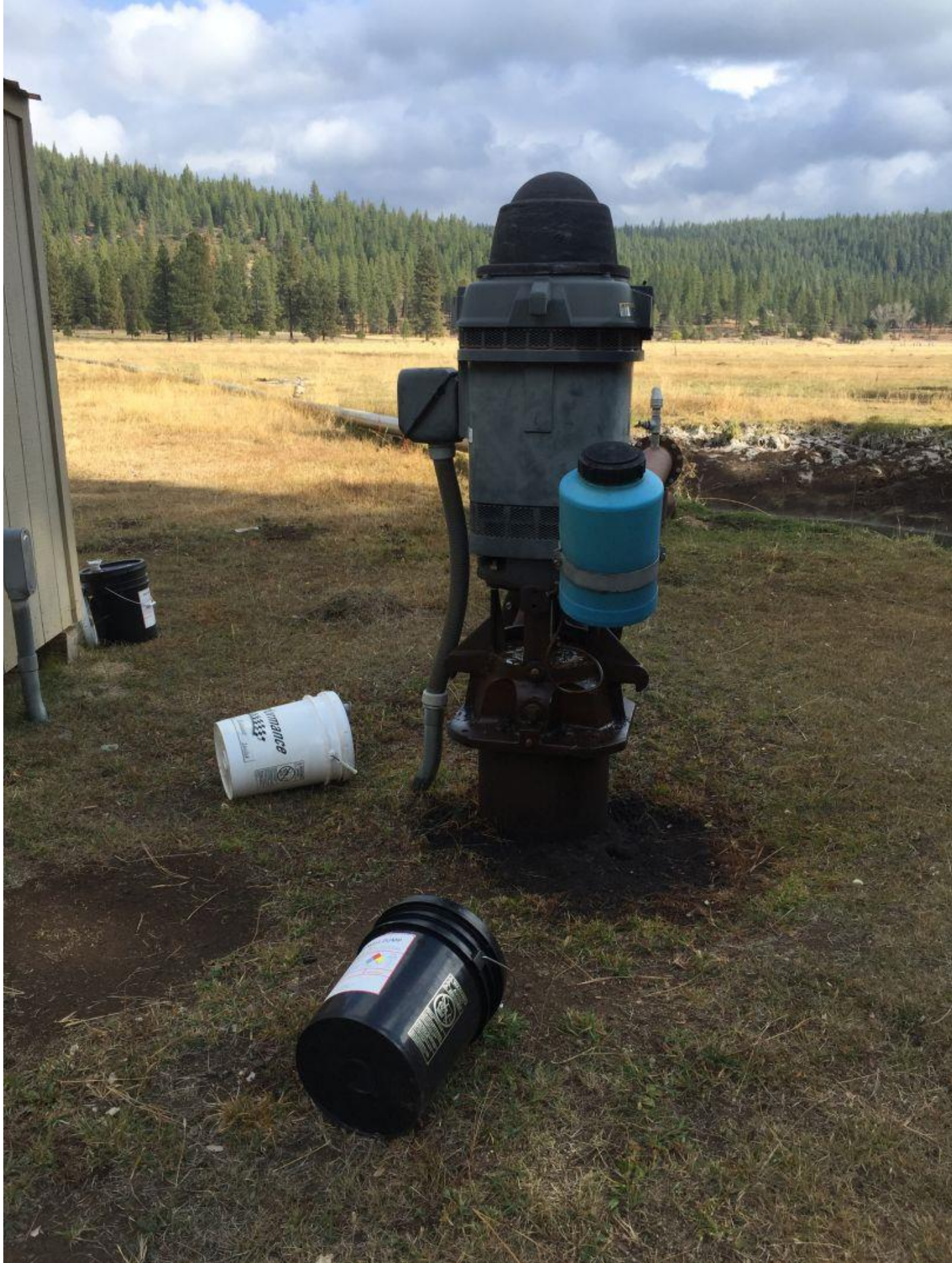
Groundwater well, pump, and shed just below Diversion 30. Capacity is likely greater than 6 cfs
