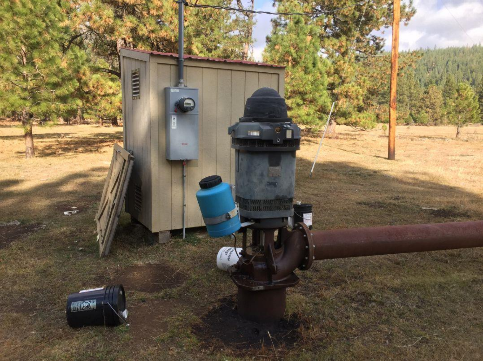
Groundwater well, pump, and shed just below Diversion 30. Capacity is likely greater than 6 cfs
