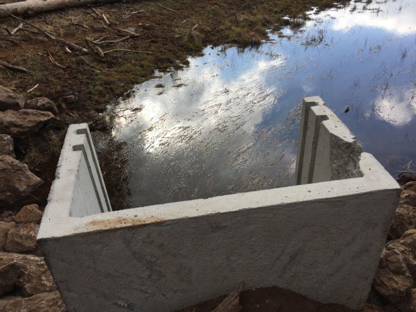
Diversion 35 bulkhead in Hemstead Dam No. 5, which serves as a 3.92-foot-wide rectangular weir box
