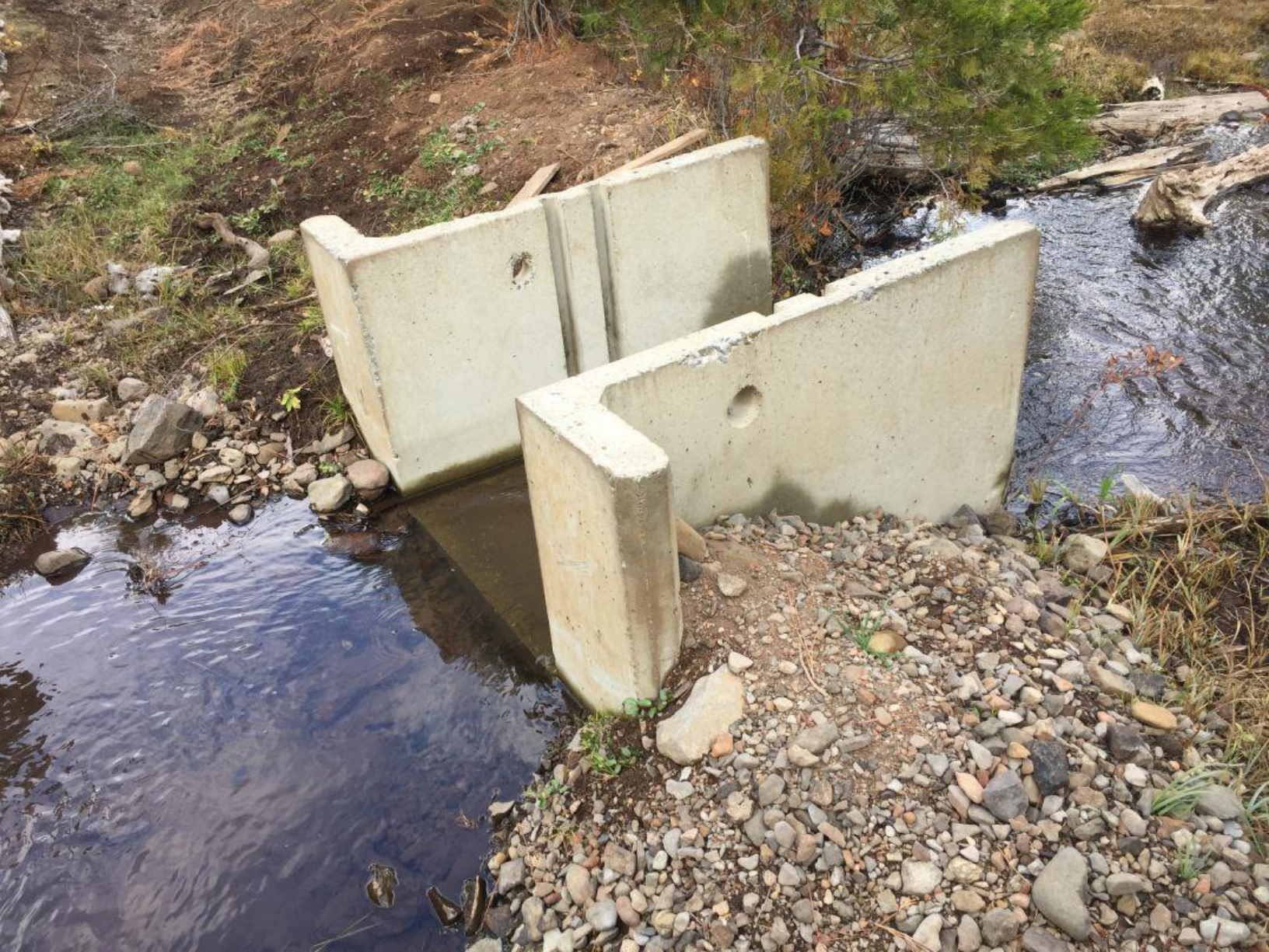
Spring from west side of the valley, between Diversions 30 and 31, showing the 2.78-foot-wide weir box
