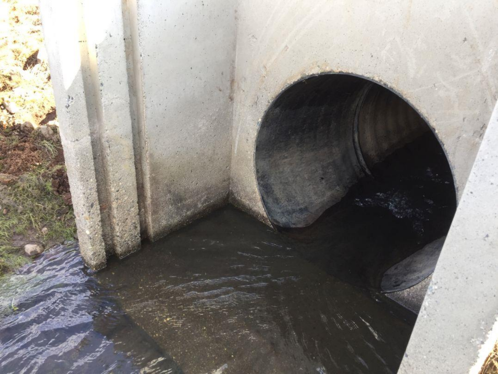
Diversion 31 bulkhead in Hemstead Dam No. 1, which serves as a 3.98-foot-wide rectangular weir box
