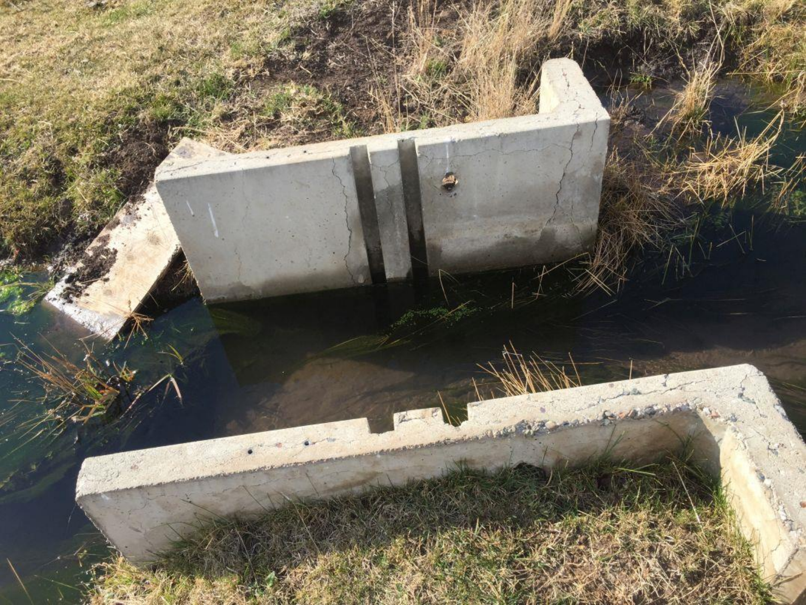
2.8-foot-wide weir box in the ditch from Diversion 30, below the dry Widow Valley Creek streambed
