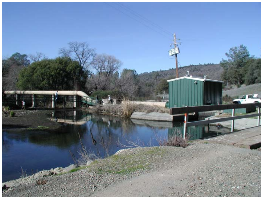
Figure 4.8-4 Asbury Pump Station
