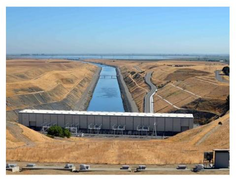
Figure 27-5: Harvey Banks Pumping Plant. Channel from the Clifton Court Forebay heads to the pumping plant and up to the Bethany Reservoir.
