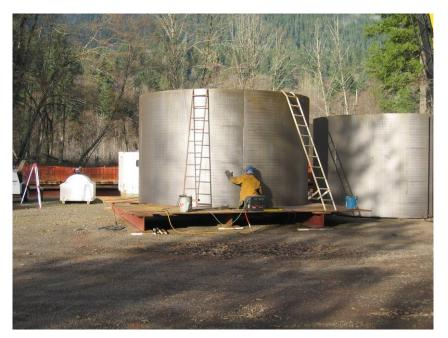
Figure 3: On-Site Fabrication of Bent Plate Steel Pipe
