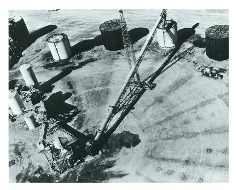
Figure 5: Ameron's On-Site Fabrication of Pre-Stressed Concrete Cylinder Pipe
