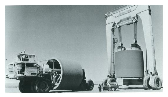
Figure 6: Ameron Used the "Pipemobile" and "Liftmobile" to Fabricate and Install 21-Foot-Diameter Pre-Stressed Concrete Cylinder Pipe On Site
