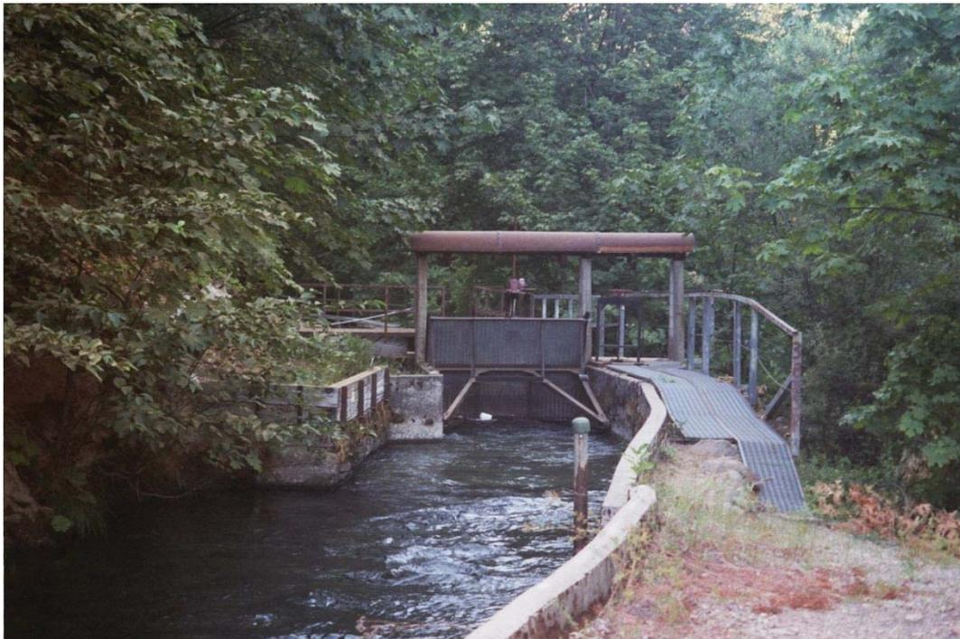
Figure 3: Hendricks Canal just downstream of Hendricks Diversion Dam: top view of works where bypass flow is released back into the West Branch Feather River. Photo by Chris Shutes.
