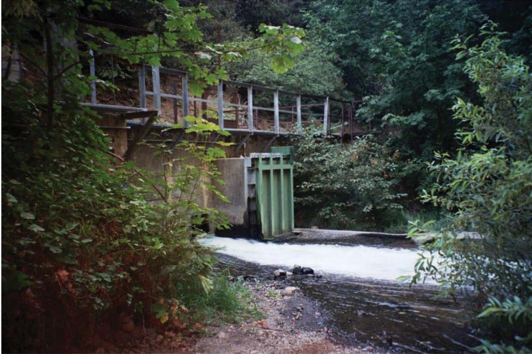
Figure 4: Hendricks Canal just downstream of Hendricks Diversion Dam: side and bottom view of works where bypass flow is released back into the West Branch Feather River. Photo by Chris Shutes.
