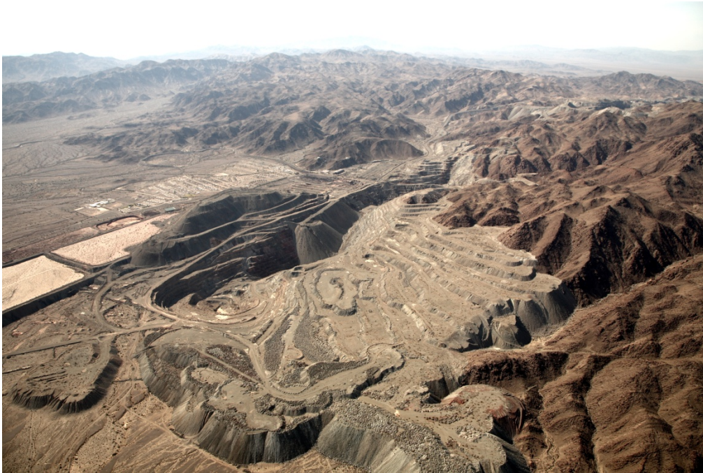
Photo 2. View towards the south, Eagle Mountain Pumped Storage Project area. Eagle Creek channel is visible in upper right of photo.
