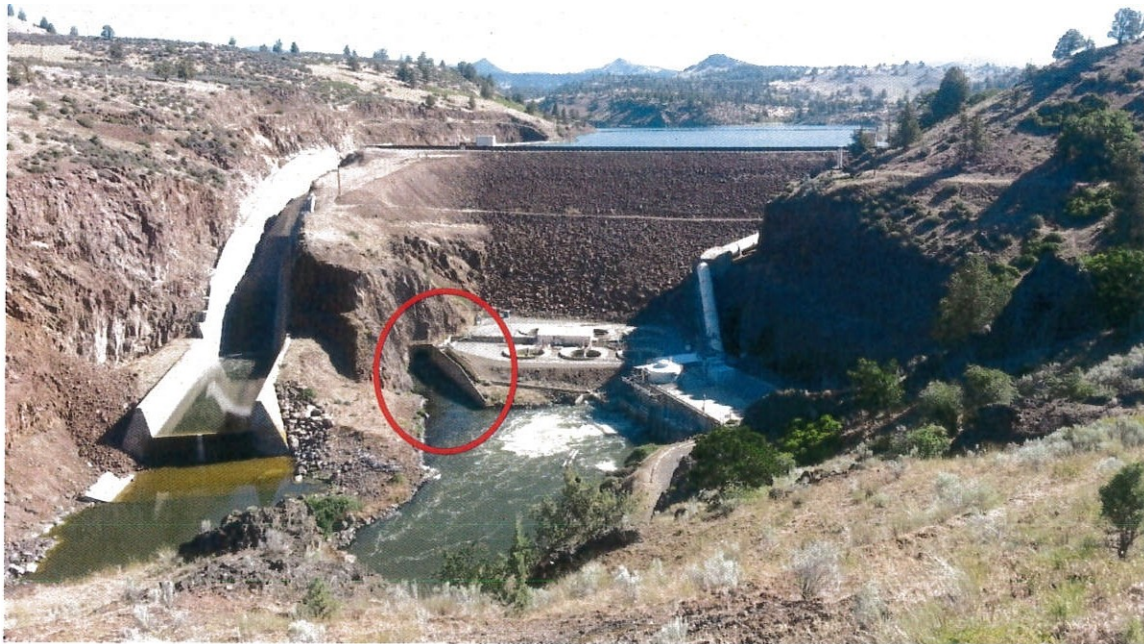
Figure 2: Low Level Outlet Discharge into Klamath River at Base of Iron Gate Dam
