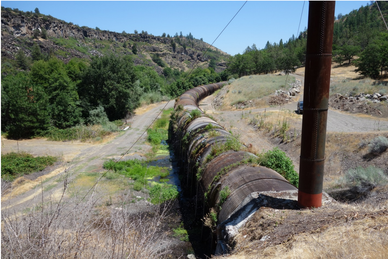
Figure 2.3-6 Copco No. 2 Wood-Stave Penstock
