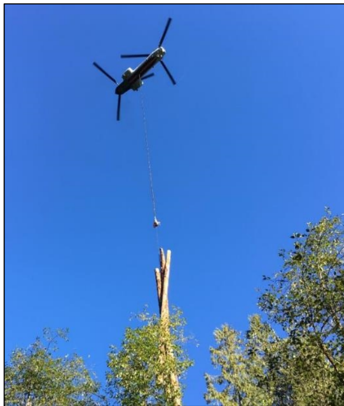
Figure 5-15 Example of LW being transported and placed with a twin rotor helicopter
