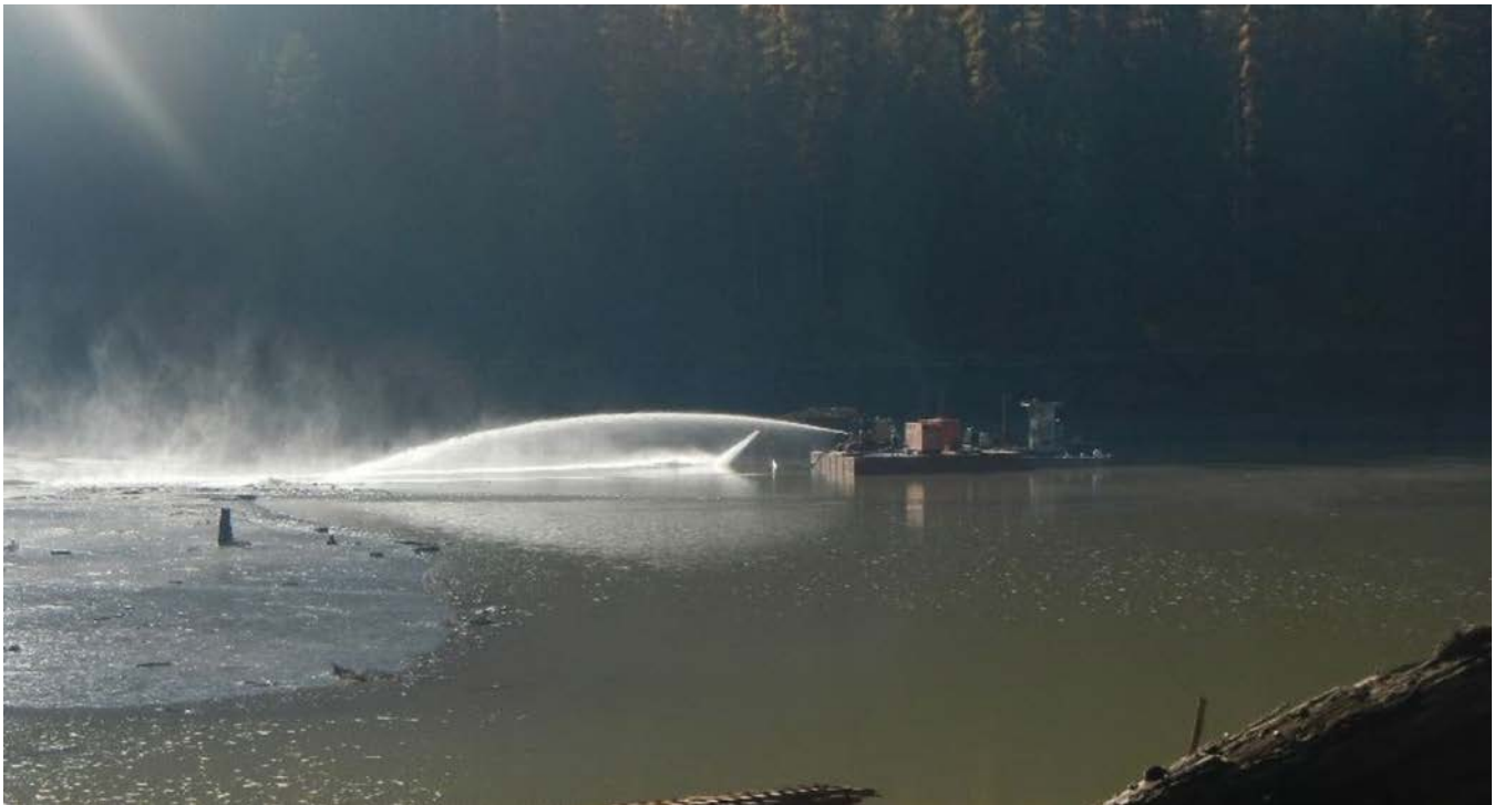
Figure 5-10 Sediment jetting on Mill Pond reservoir using a barge and excavator with pump and spray nozzles to maximize stored sediment erosion during reservoir drawdown (photo from Envirocon)
