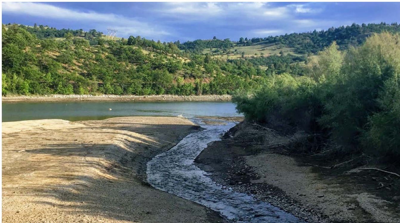
Figure 5-11 Jenny Creek tributary on Iron Gate reservoir with reservoir drawn down approximately 20 ft showing deposition and small delta where it intersects with reservoir in 2018
