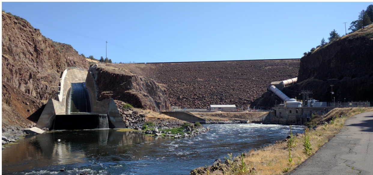
Figure 2.4-2 Iron Gate Dam, Spillway (left), and Powerhouse (right)
