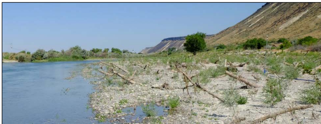
Figure 5-13 Example of restored floodplain area six months after construction in an arid climate showing new vegetation and wood roughness elements that provide habitat complexity and immediate, large scale roughness
