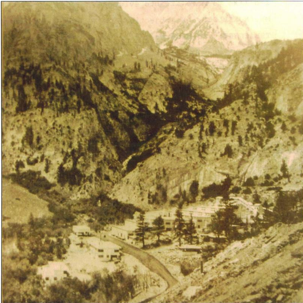
Figure 11.1.3. Concentrating and chemical treatment plant of U.S. Vanadium Corp. at junction of Pine and Morgan Creeks, elevation 7,700 ft. (Photograph from Engineering and Mining Journal , November 1941: 72.) This photograph, looking southwest, was taken from Morgan Creek Road leading to the upper mining area.
