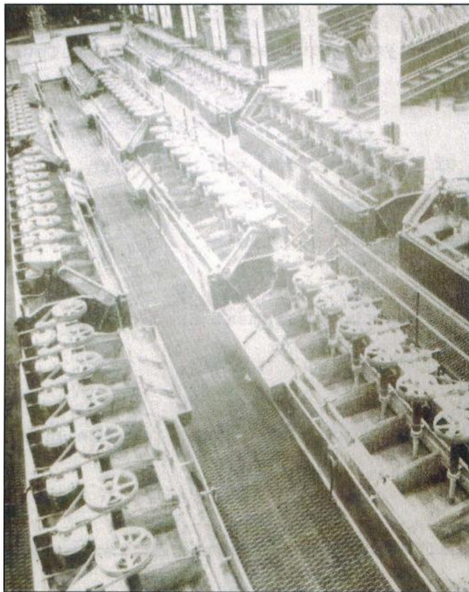
Figure 11.1.10. Flotation Section at Pine Creek uses M.S. machines, makes copper, molybdenum, and scheelite concentrate (Photograph from Engineering and Mining Journal, May 1951:83).
