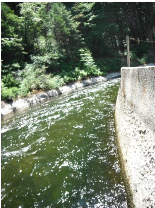
Figure 5. View of escape ramp taken upstream near edge of canal, showing escape ramp is not visible on approach.
