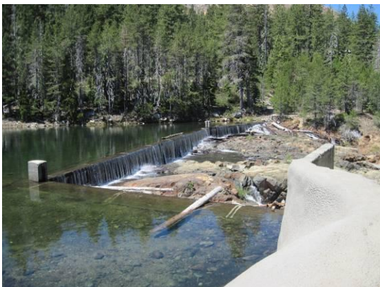
Picture - Sawmill Spillway (unsafe crossing)
