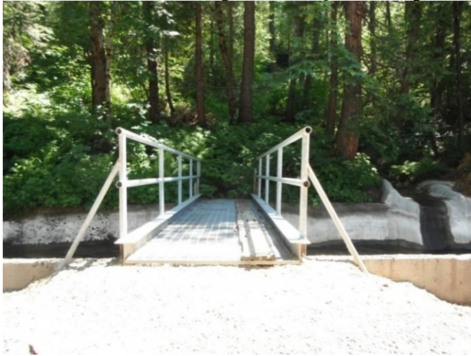
Figure 3. Drum Canal Crossing (FS73/GPSID YDWMDC037). Technical Memo 4-2 metadata notes “planks placed over grate.” The current 9-inch width of planks does not meet recommended widths (>3-10M) (Clevenger and Huijser 2011, p. 110, 140) for crossings.
